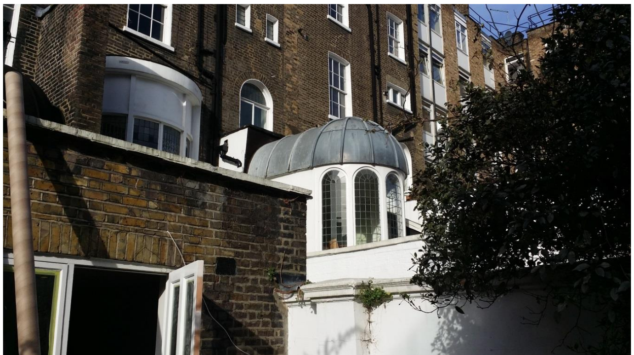
Other structures on the rear of the terrace
